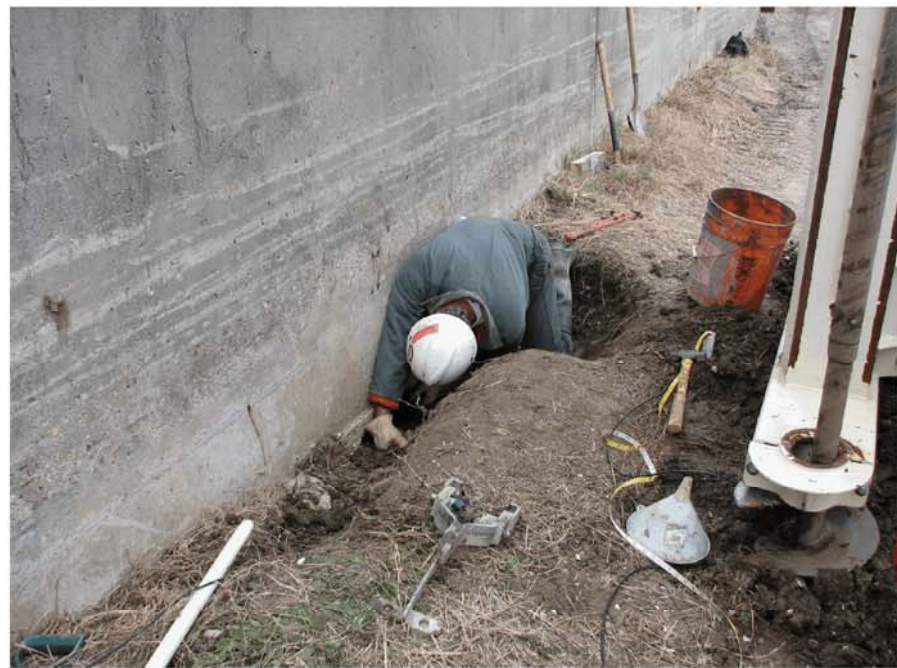
Photo 9 - IHNC 3-lb Impulse hammer impacts to sheet pile on canal side at Station 17+11
